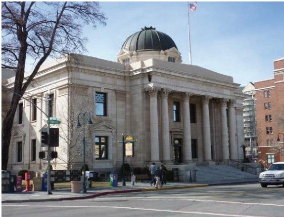
Washoe County Courthouse
